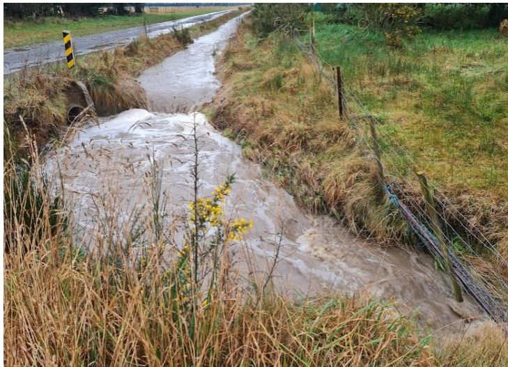
Image 3 Scotts Road flow when in very minor rain event – significant flow going into shingle pit at Thwaites/Scotts intersection, keeping water away from Hororata
